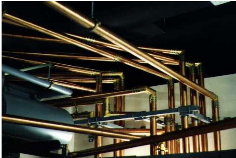
RF plumbing at the Empire State Building
